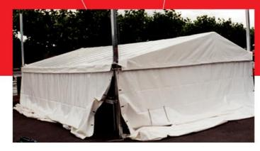
After the support and roof structure has been installed and the tarpaulins for the roof and sides have been attached, the roof structure is brought into position using 4 hand winches.
